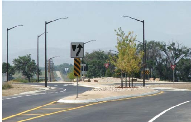
Exhibit 14.12. Example of undesirable blockage of stopping sight distance on roundabout approaches.
