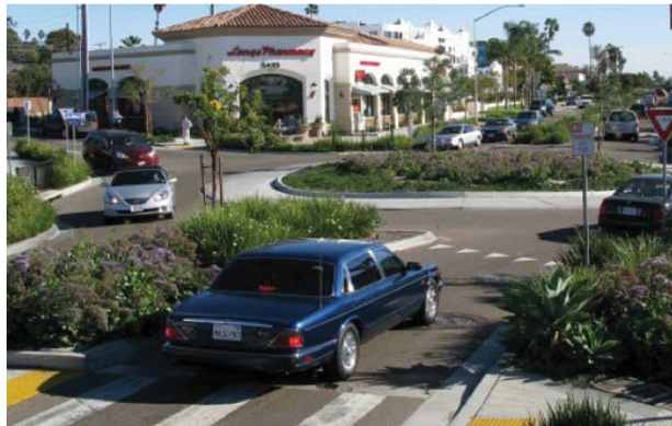
Exhibit 14.13. Example of undesirable blockage of intersection sight distance at roundabout entry.
